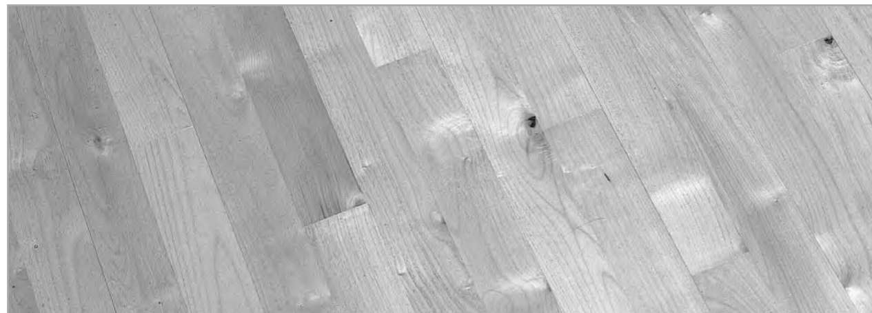
Narrow board sycamore hardwood floor laid with quick clip system
