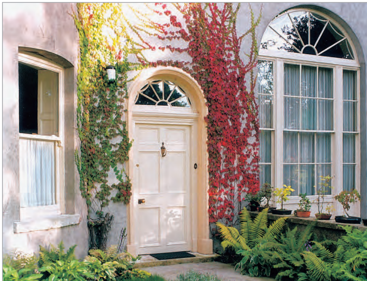
Victorian replacement and original Georgian joinery forms part of the history of this 1732 estate house in the National Botanic Gardens.
