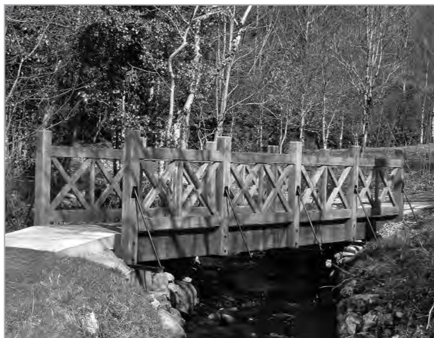
Fig. A 16.2.5.4 Oak bridge at Lough Gill, Sligo.
