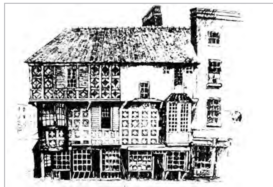
Fig. A 15.1 An historic illustration of the last recorded urban timber-framed historic building in Ireland. Note the angle posts and jettying of the upper floor, the various expressions of bracing, and decorative quatrefoil panelling on the second and third floors similar to extant buildings in Lancashire, Essex, and Shropshire in Britain. This illustration shows a shop and house built by Nicholas Bathe on the corner of Shop St. and Laurence St. in Drogheda, Co. Louth. It was demolished in 1824.
