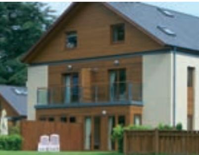
Allowing moulded cladding to acclimatise to its end use environment conditions prior to installation will also reduce movement after installation.
