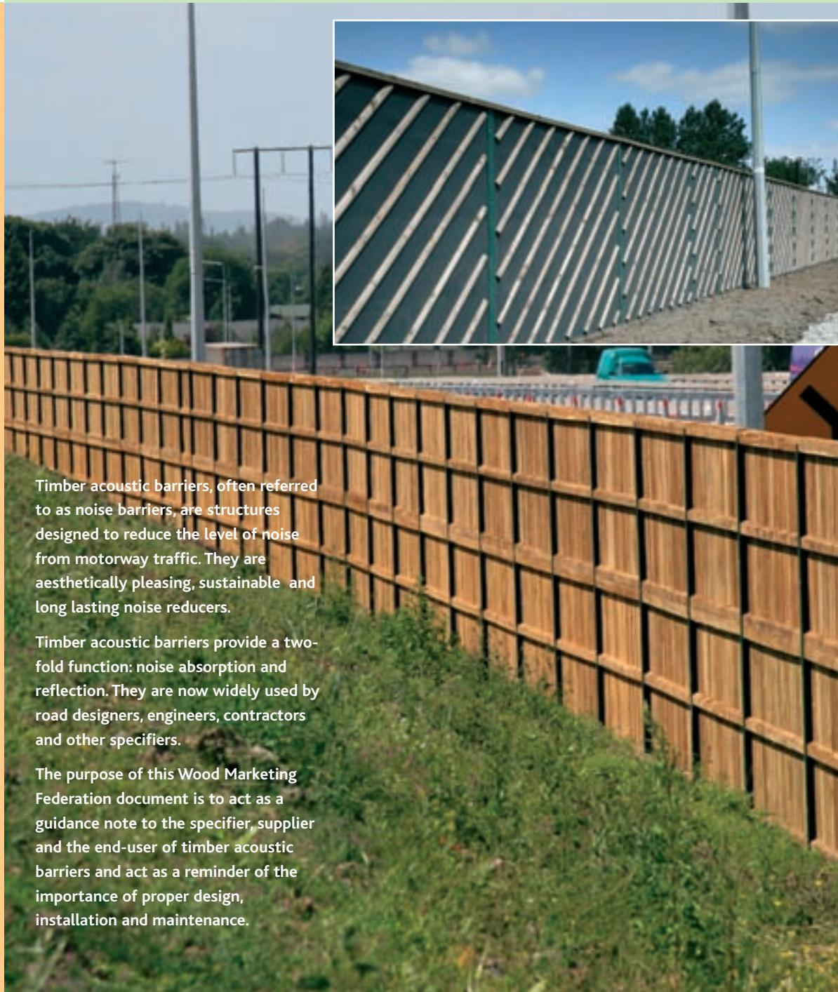
Timber acoustic barriers, often referred to as noise barriers, are structures designed to reduce the level of noise from motorway traffic. They are aesthetically pleasing, sustainable and long lasting noise reducers.
