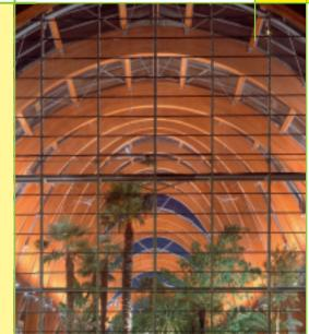
Wood has been an important construction material for centuries. Today, it is engineered to provide even greater strength qualities. Engineered wood includes glulam which is used in sports' arenas, glasshouse supports and concert halls.
